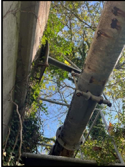
Photo 7: Abutment No. 2 – Detached Utility Hanger
