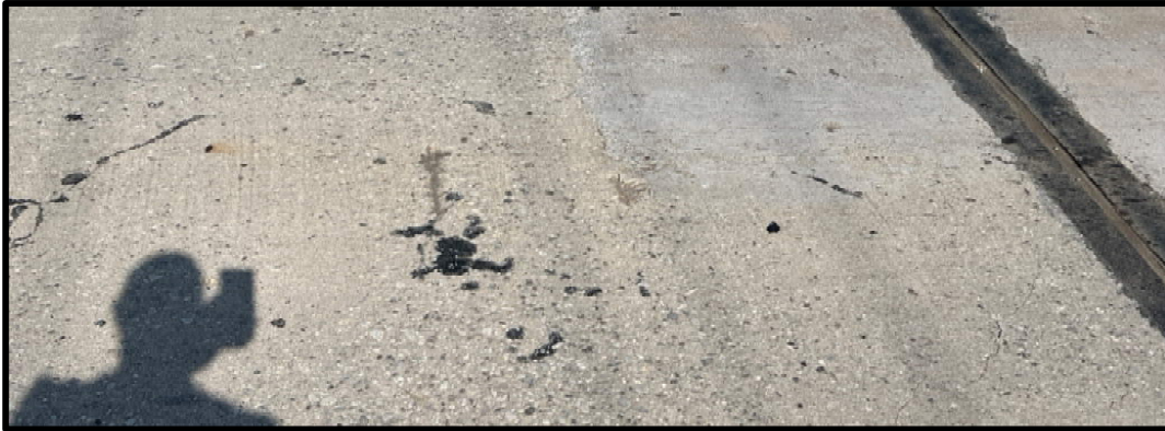
Photo 37: Span 8 above Bent 6, Top Deck – Exposed Rebar
