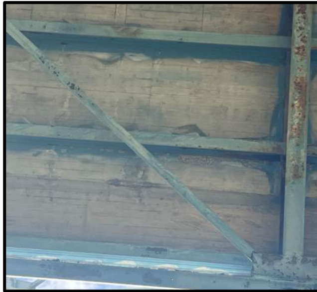
Photo 47: Truss 3, Bottom Deck Section 25 – Exposed Rebar, Spalling, Corrosion, Paint Peeling
