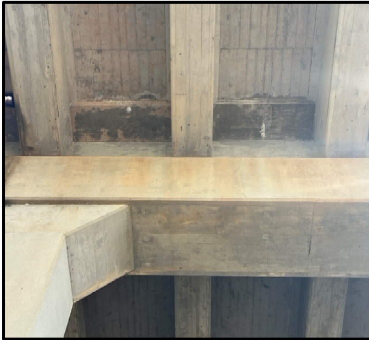
Photo 55: Span 9, Beam B & C & D – Efflorescence near Bent 7
