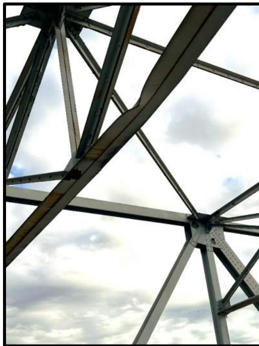
Photo 20: Sway Frame 4 – Collision Damage near Quarterspan of Bottom Right Chord
