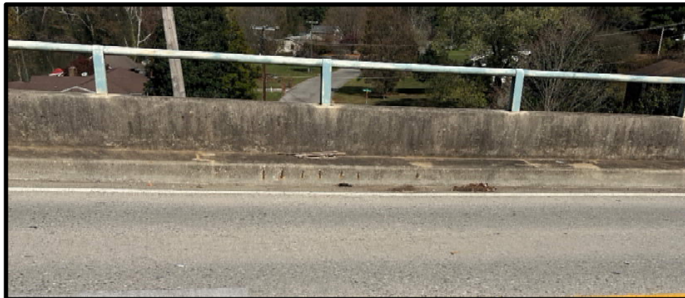
Photo 36: Span 8, Sidewalk – Exposed Rebar and Spalling Left Shoulder
