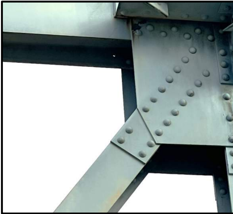
Photo 25: Truss 2, Left – U15L Missing Rivet
