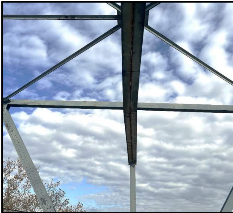
Photo 30: Sway Frame 24 – Misalignment
