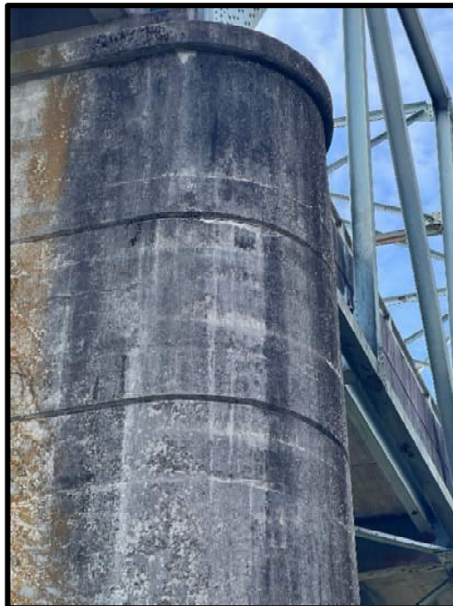
Photo 10: Pier No. 4 – Spalling and Popouts
