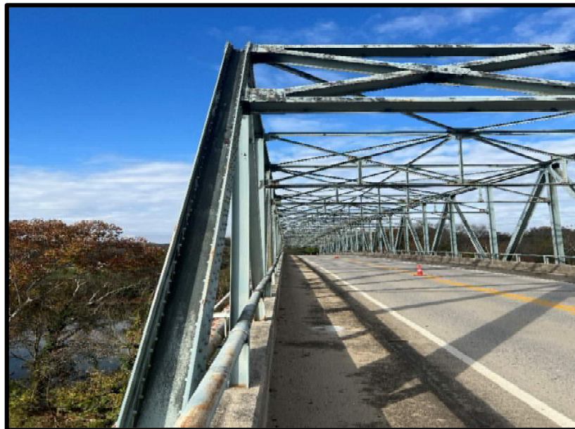
Photo 32: Truss 3, Portal – Dirt Buildup in U25R-L26R
