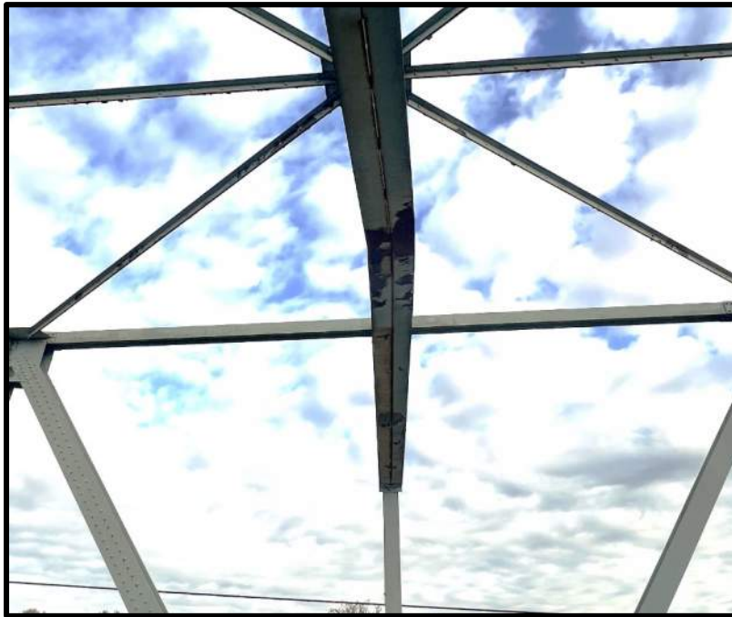
Photo 23: Sway Frame 6 – Misalignment
