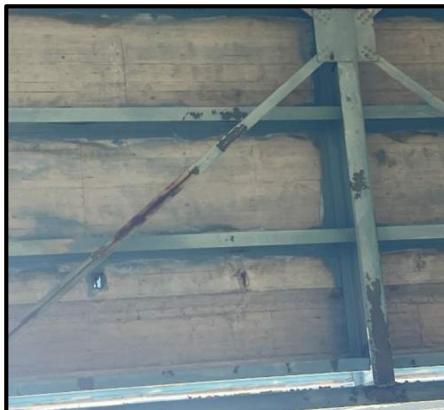
Photo 44: Truss 3, Bottom Deck Section 22 – Exposed Rebar, Spalling, Corrosion, and Paint Peeling
