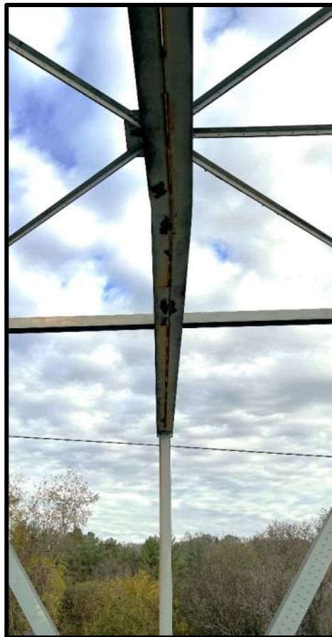
Photo 18: Sway Frame 2 - Misalignment
