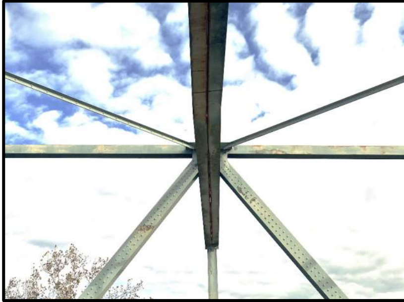
Photo 27: Sway Frame 23 – Misalignment
