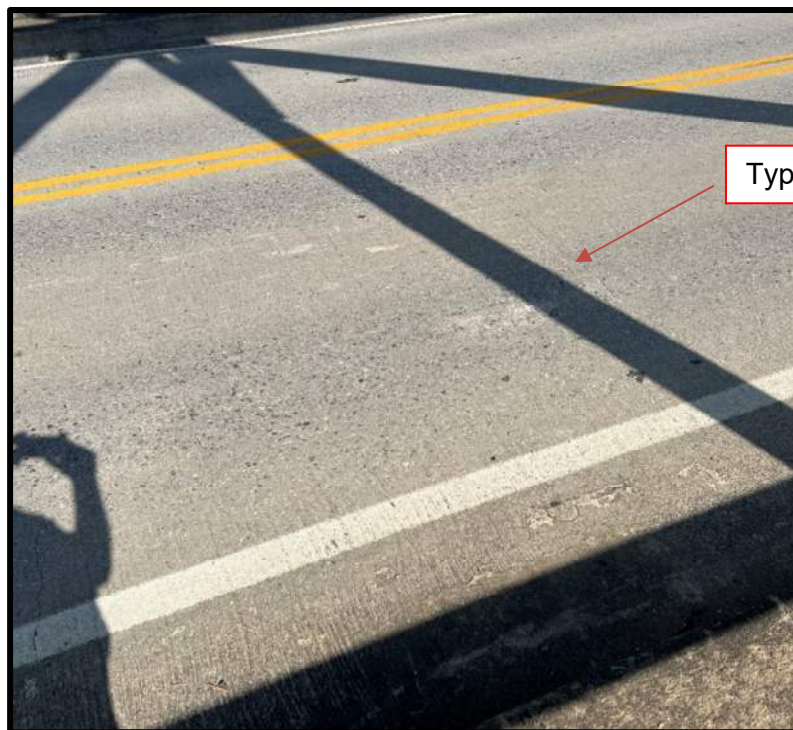
Photo 34: Top Deck – Abrasion and Cracking (typ. across bridge)
