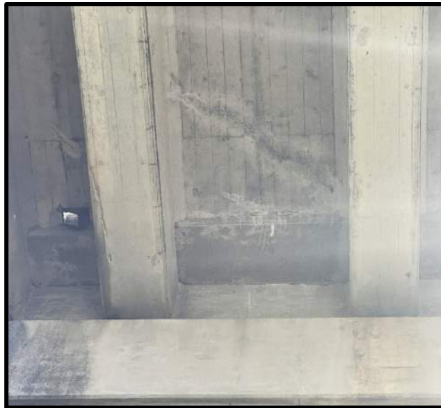
Photo 50: Span 7, Beam B & C – Crack and Efflorescence near Bent 5
