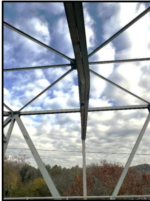
Photo 21: Sway Frame 4 – Misalignment
