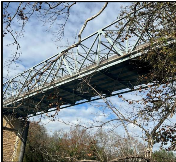
Photo 40: Truss 2, Bottom Deck Section 9-18 – General Overview and Corrosion, Spalling, Exposed Rebar, Paint Peeling
