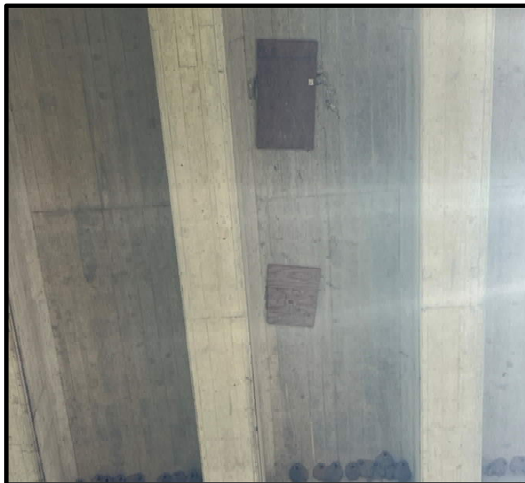
Photo 52: Span 8, Beam C & D – Patched Spalls with Plywood near Bent 5
