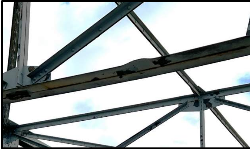
Photo 17: Sway Frame 2 – Collision Damage at Quarterspan of Bottom Right Chord
