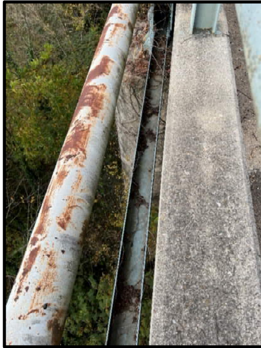
Photo 11: Debris Buildup in Lower Chord L0R-L1R (typ.)
