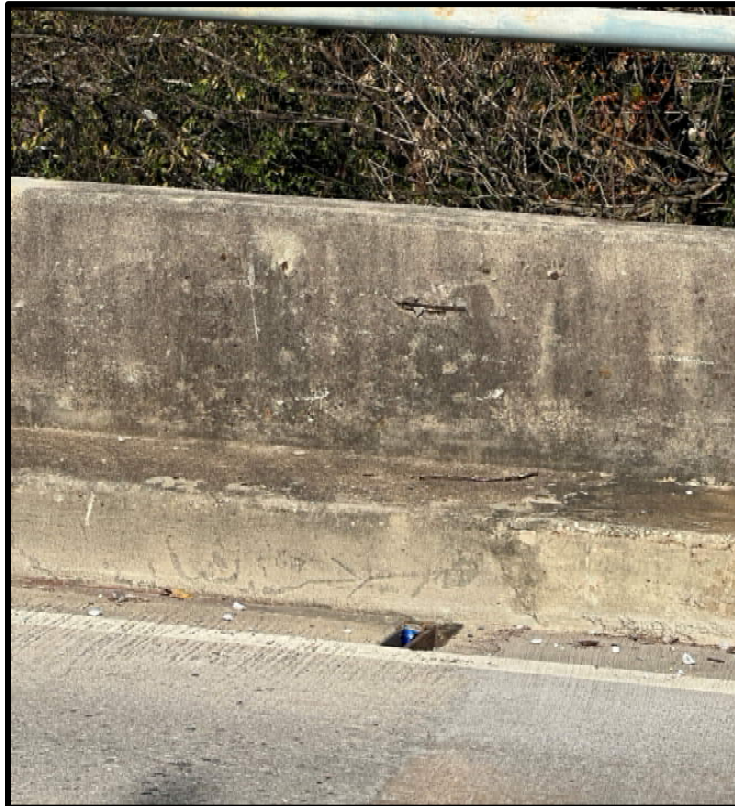
Photo 38: Span 9 at Bent 7, Sidewalk – Exposed Rebar
