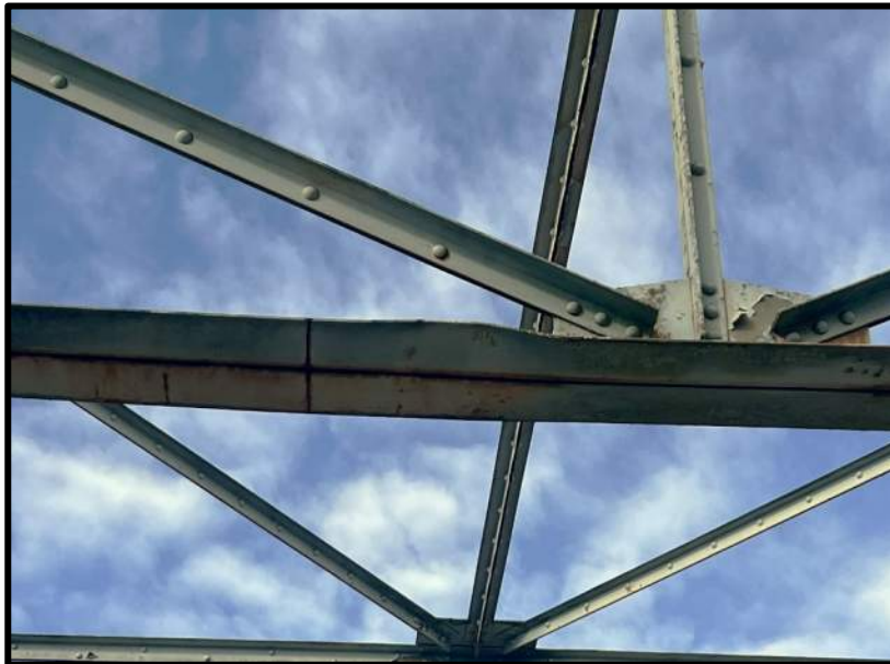
Photo 26: Sway Frame 23 – Collision Damage near Middle Web on Bottom Right Chord
