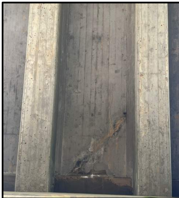
Photo 56: Span 10, Beam B & C – Crack near Bent 7
