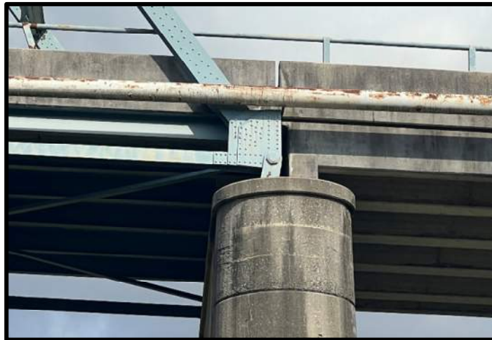
Photo 48: Truss 3, Bearing Device – Tilted East
