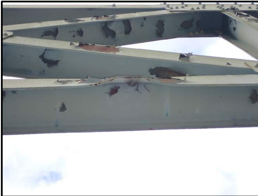
Photo 16: Truss 1, Portal – Collision Damage at Bottom Right Chord
