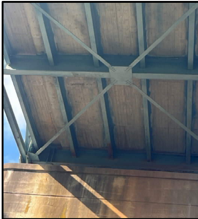
Photo 42: Truss 3, Bottom Deck Section 19 – Exposed Rebar, Spalling, Corrosion, and Paint Peeling
