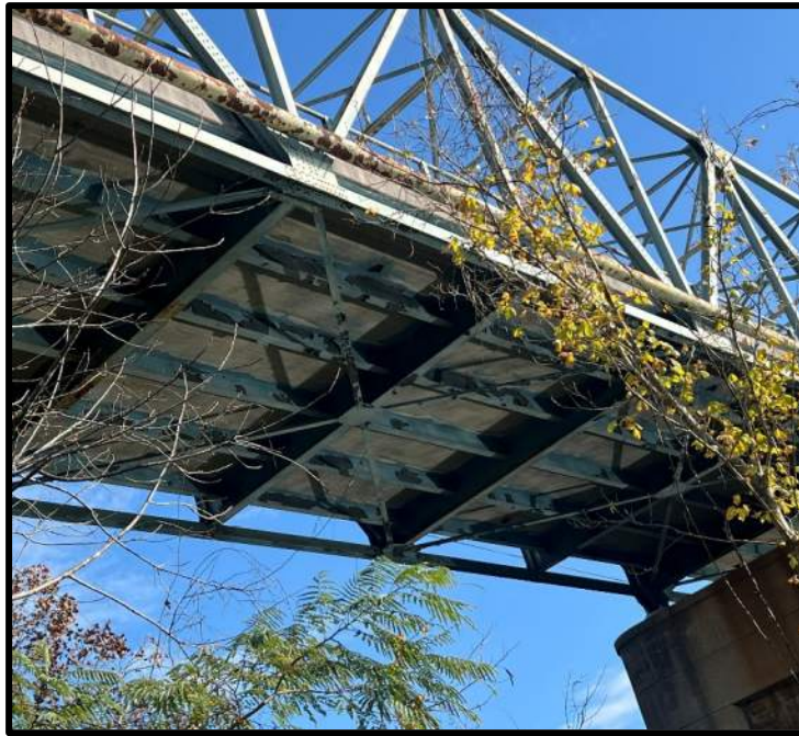
Photo 39: Truss 1, Bottom Deck Section 1-8 – General Overview and Corrosion, Spalling, Paint Peeling
