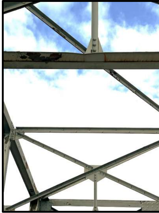
Photo 19: Sway Frame 3 – Collision Damage near Midspan of Bottom Right Chord
