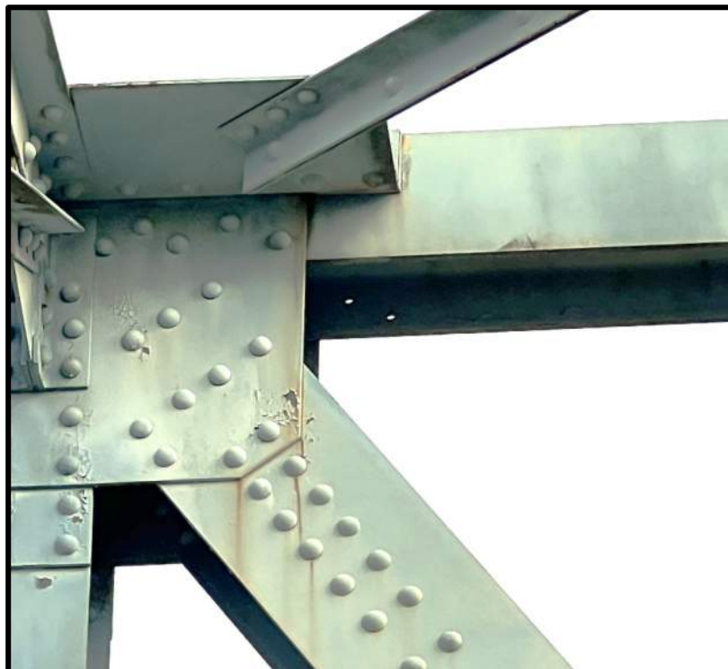
Photo 24: Truss 2, Left – U13L Missing Rivets
