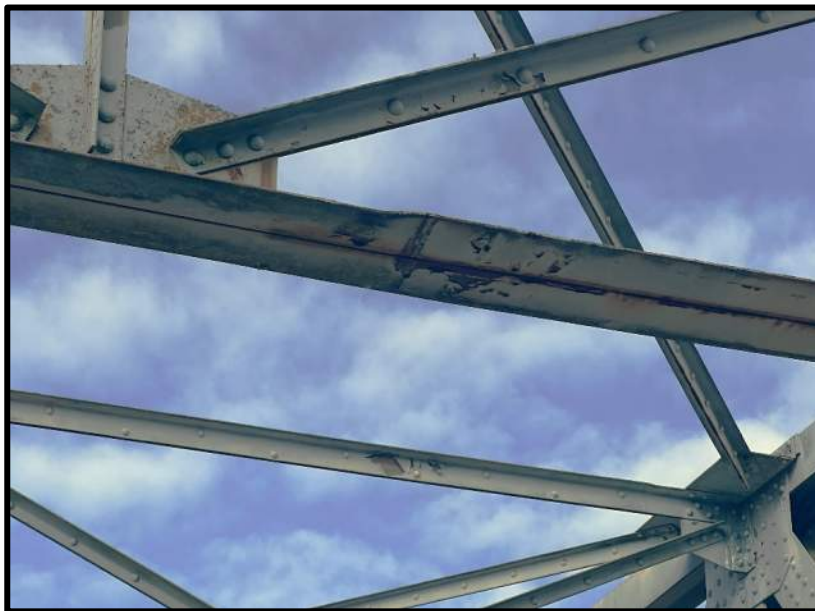
Photo 28: Sway Frame 24 – Collision Damage near Middle Web on Bottom Left Chord
