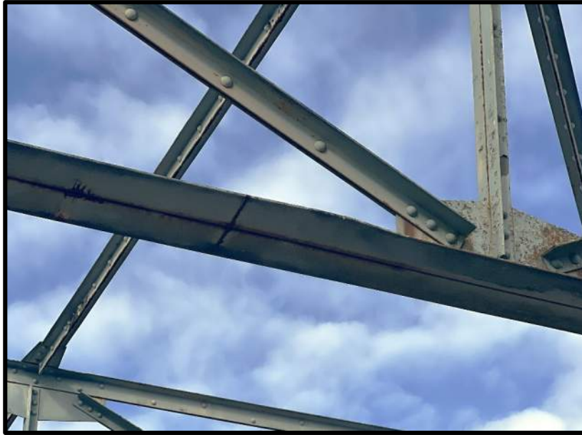
Photo 29: Sway Frame 24 – Collision Damage near Middle Web on Bottom Right Chord
