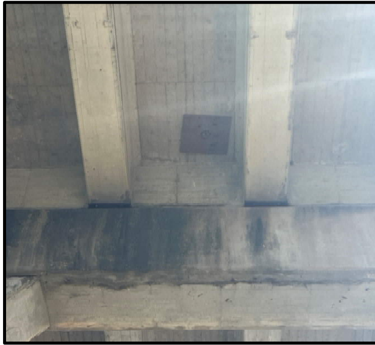
Photo 53: Span 8, Beam C & D – Patched Spall with Plywood near Bent 6
