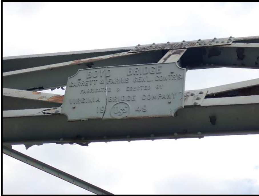
Photo 15: Truss 1, Portal - Sign Cracked Through
