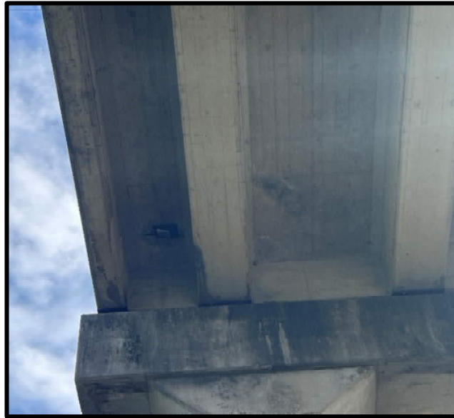
Photo 51: Span 8, Beam A & B – Spall Around Drain near Bent 6, Beam B & C – Crack near Bent 6
