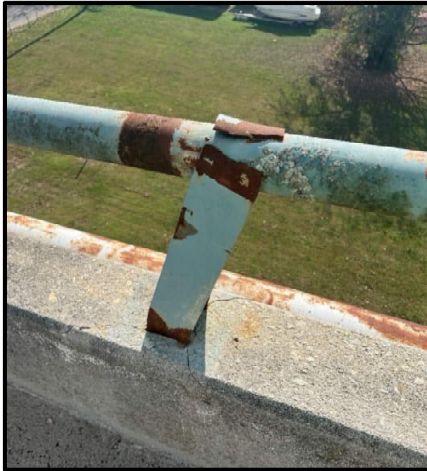
Photo 35: Railing above L24R-L25R – Corrosion, Cracking and Misalignment
