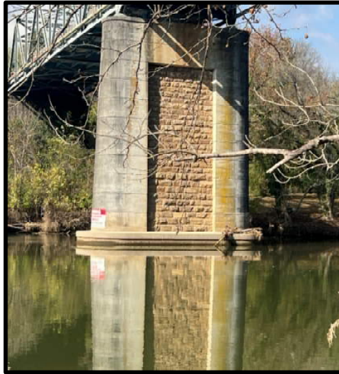
Photo 9: Pier No. 3 – Drift Build-up (typ.)
