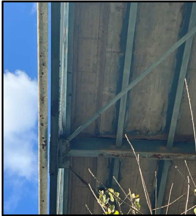
Photo 43: Truss 3, Bottom Deck Section 21 – Exposed Rebar, Spalling, Corrosion, and Paint Peeling
