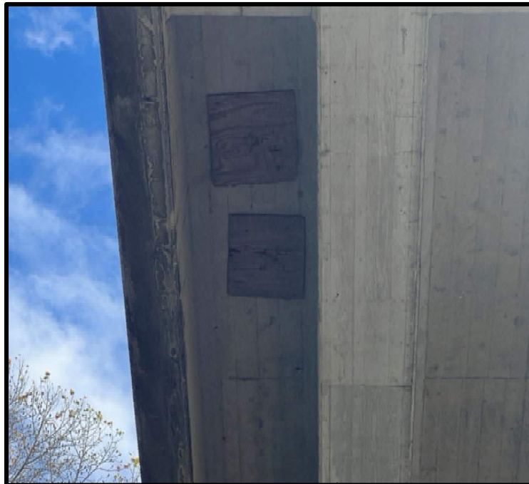
Photo 54: Span 9, Beam A & B – Patched Spalls with Plywood near Bent Midspan
