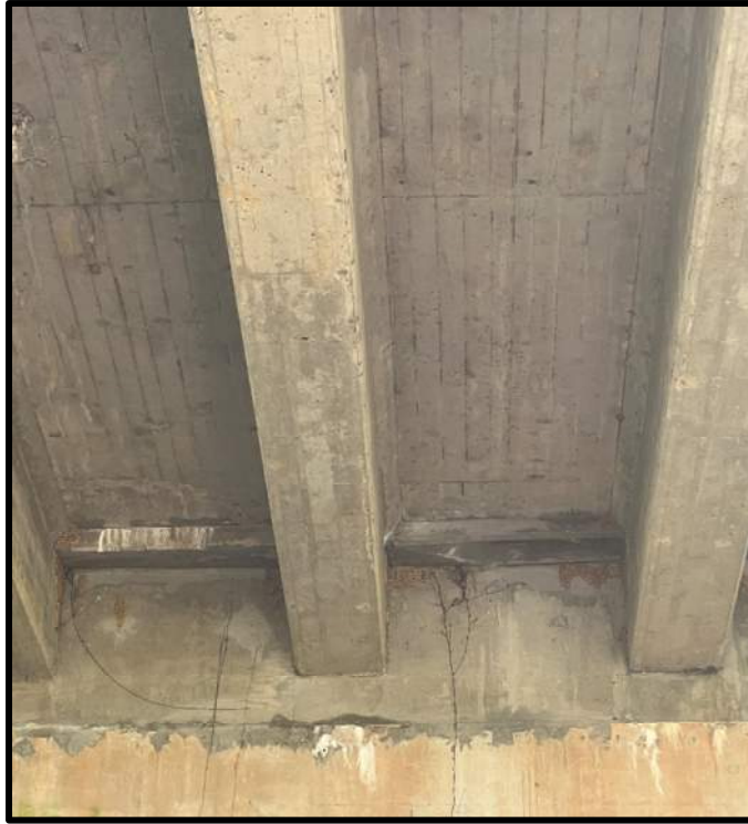
Photo 57: Span 10, Beams B & C & D & E – Efflorescence near Abut. 2
