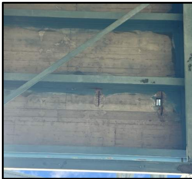
Photo 46: Truss 3, Bottom Deck Section 24 – Exposed Rebar, Spalling, Paint Peeling
