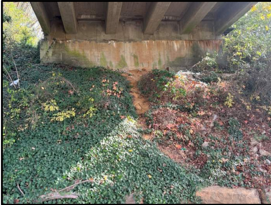
Photo 5: Abutment No. 2 (Eastern) – Vegetation and Efflorescence Observed
