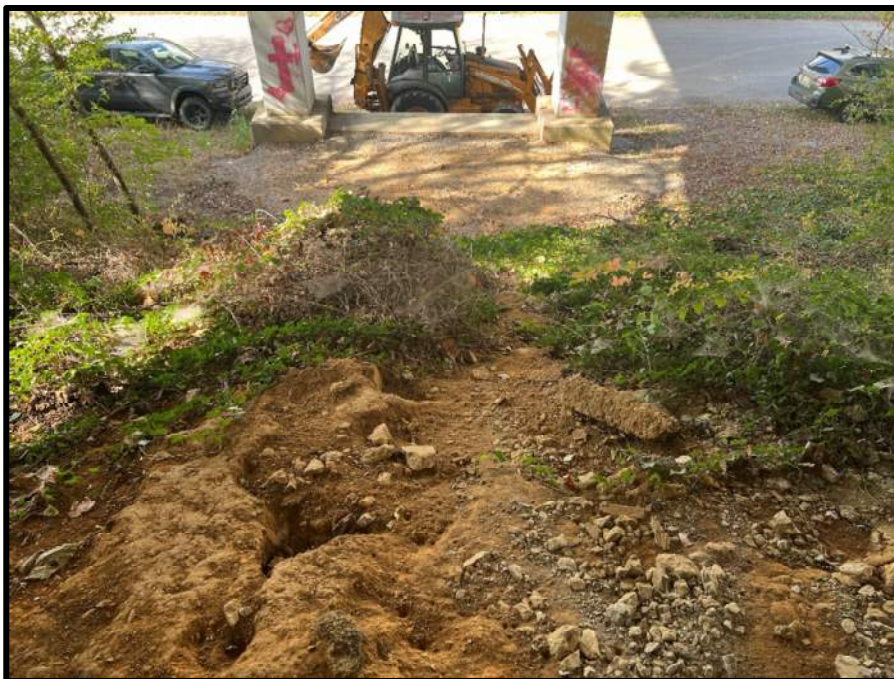
Photo 6: Abutment No. 2 (Eastern) – Slope Erosion Observed
