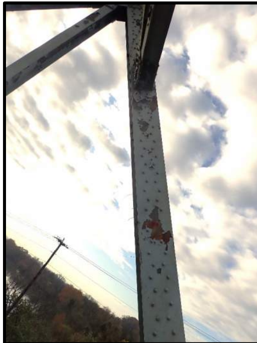
Photo 12: Truss 1, U1R-L0R Corrosion and Paint Flaking (typ. across bridge)
