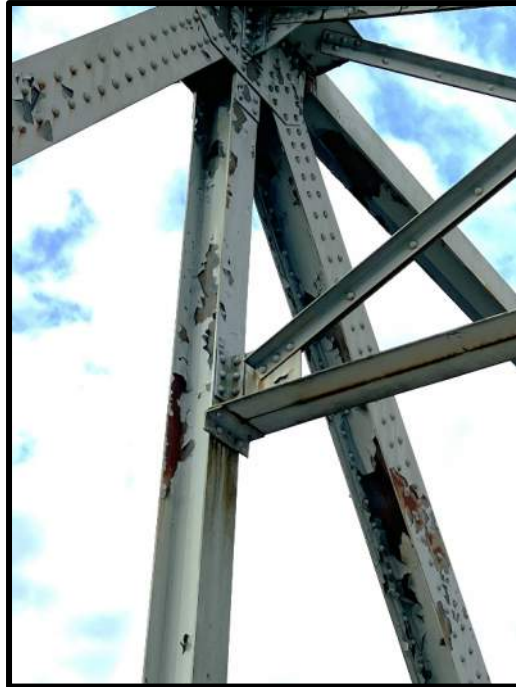
Photo 13: Truss 1, U3R-L3R Corrosion and Paint Flaking (typ. across bridge)
