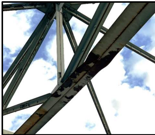
Photo 22: Sway Frame 6 – Collision Damage near Middle Web on Bottom Right Chord
